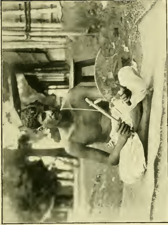
Fig. 2. Sharpening an engraving saw, Dinajpur.
